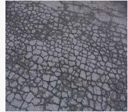
Alligator Cracking
