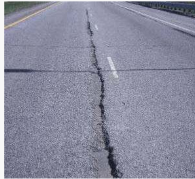
Transverse or Longitudinal Cracking
