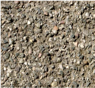
Weathering or Raveling
