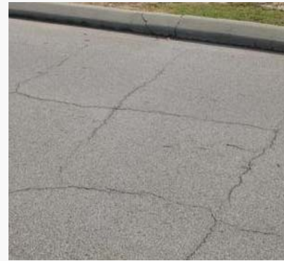
Block Cracking
