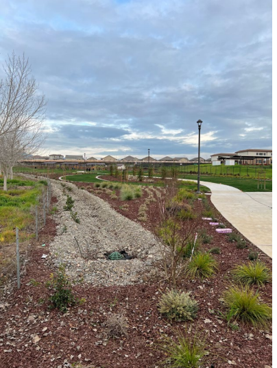
Photo 6 (pictured right) looking east from Fairview Rd. Rock placed in the swale with fabric filters below atrium grates. Bark and landscaping for ground cover.
