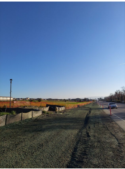
Photo 7 (pictured left) looking east from edge of pavement on Fairview Rd. Rock placed in the swale with fabric filter below atrium grate, loose soil has been sprayed with Hydroseed and silt fence has been placed for erosion and sediment control. Bark and landscaping for ground cover.
