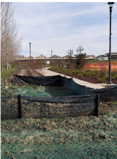
Photo 7 (pictured left) looking east from edge of pavement on Fairview Rd. Rock placed in the swale with fabric filter below atrium grate, loose soil has been sprayed with Hydroseed and silt fence has been placed for erosion and sediment control. Bark and landscaping for ground cover.
