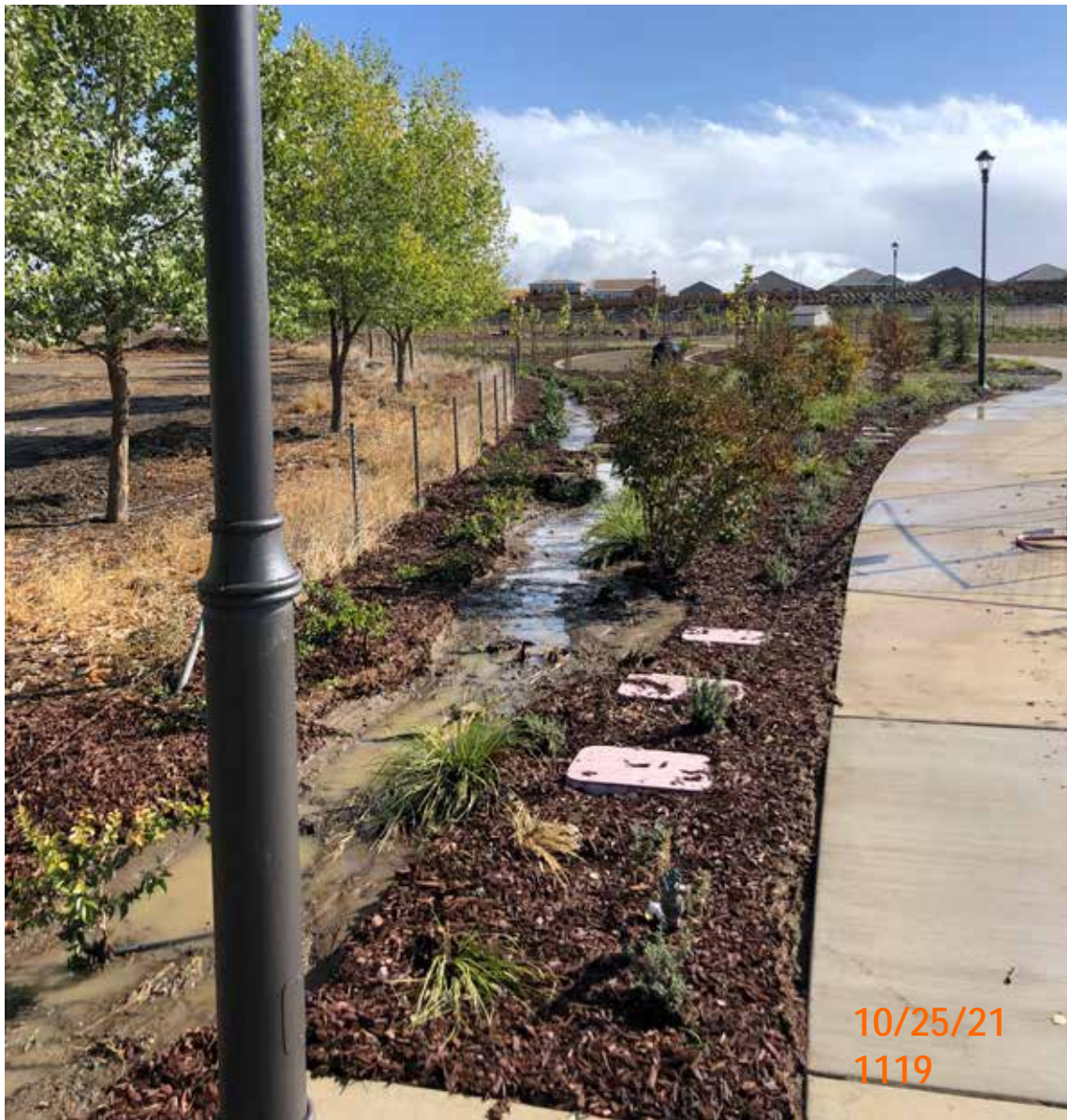
Photo 6. Looking east from Fairview Rd., south of Photo 5. Channelized flow from stormwater discharge from the community park and upland source areas.
