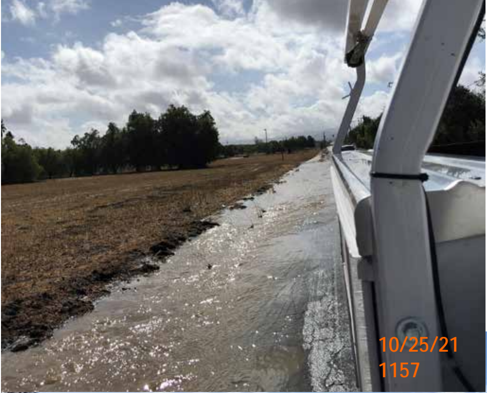
Photo 11. Looking south, edge of pavement on Fairview Rd. at location of Photo 9. Turbid water discharge from Santana Ranch Basin A and construction site.
