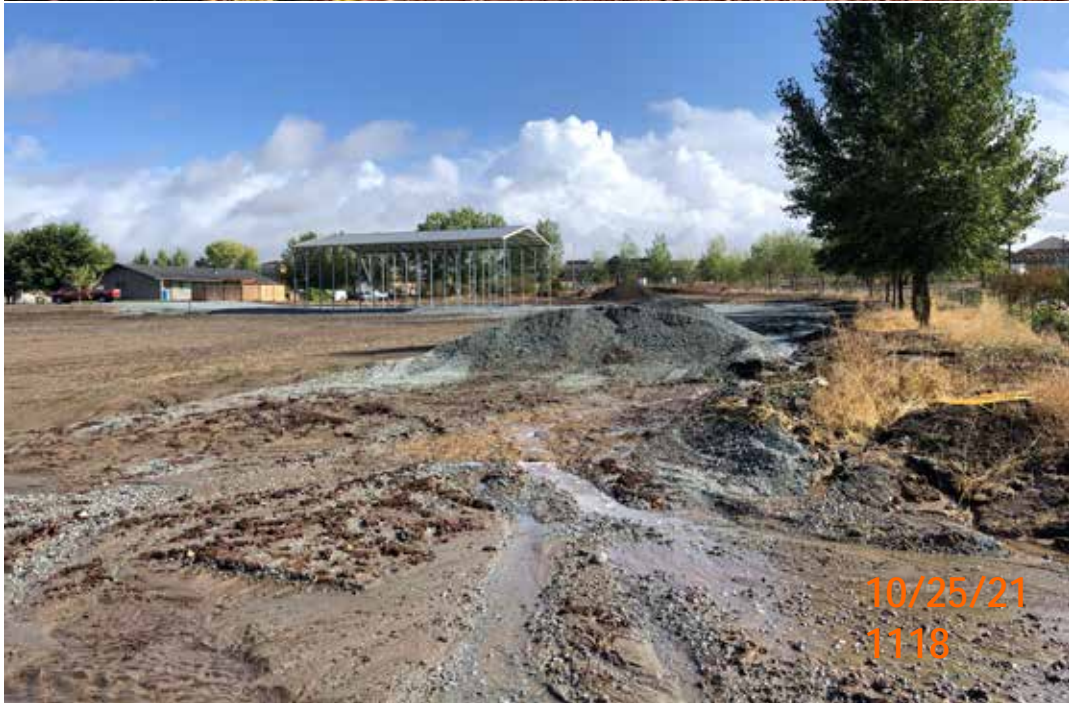
Photo 5. Look east from Fairview Rd., concentrated flow and anastomosing channels formed by discharge from community park and upland areas.
