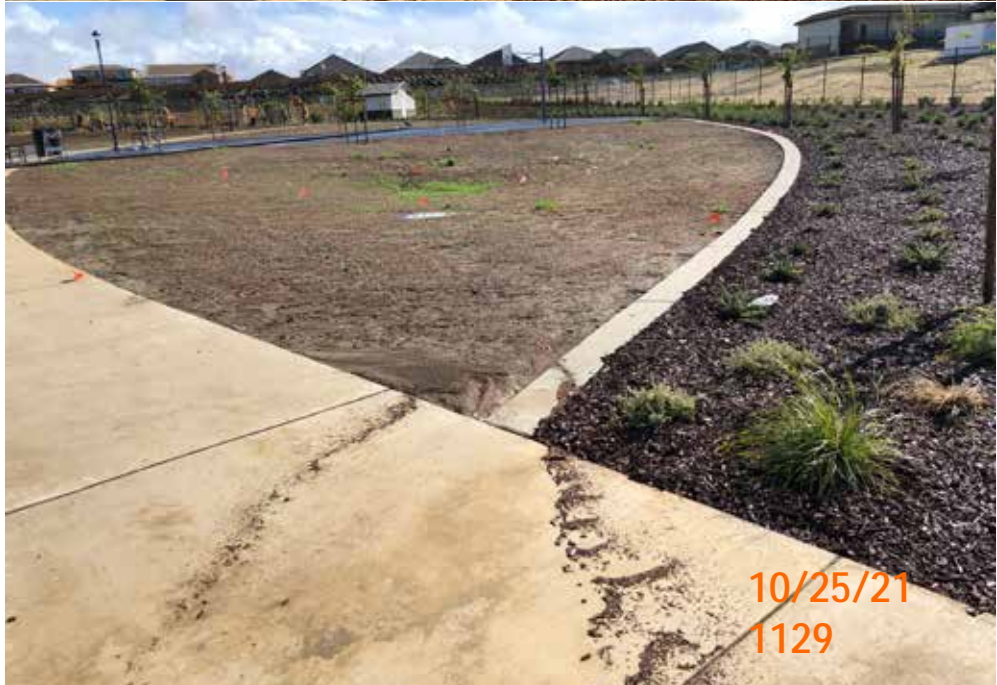
Photo 2. Community park area west of basketball court; note evidence of sheet flow across bare ground.
