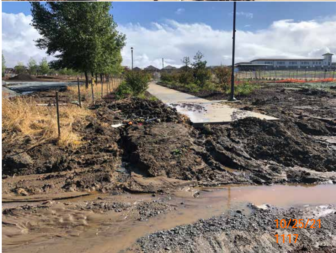
Photo 7. Looking east from edge of pavement on Fairview Rd., downstream of photo 6. Lack of erosion and sediment controls.
