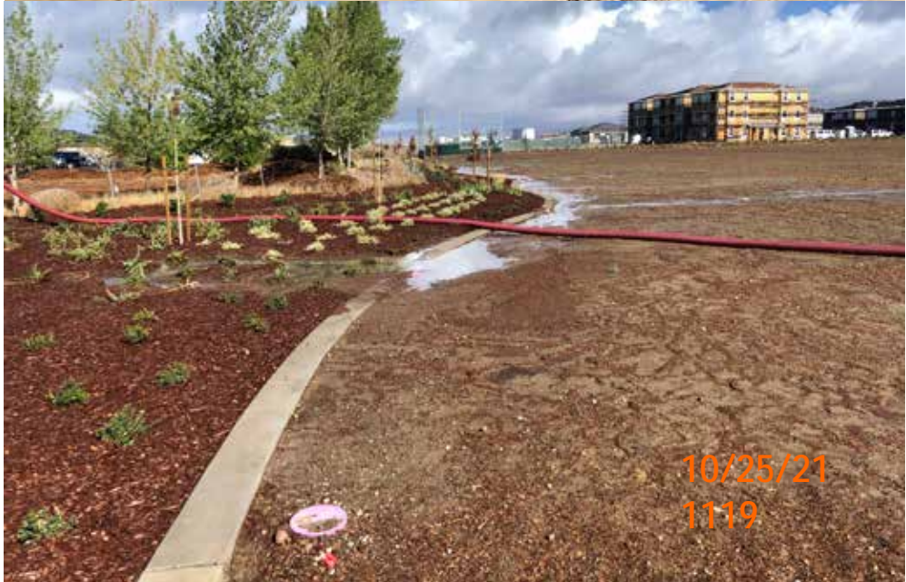
Photo 3. Community park boundary, Cal Fire to left; note sheet flow features across bare ground and concentrated flow occurring at edge strip. 4 to 6-inch hose in photo was used for pneumatic application of wood mulch.
