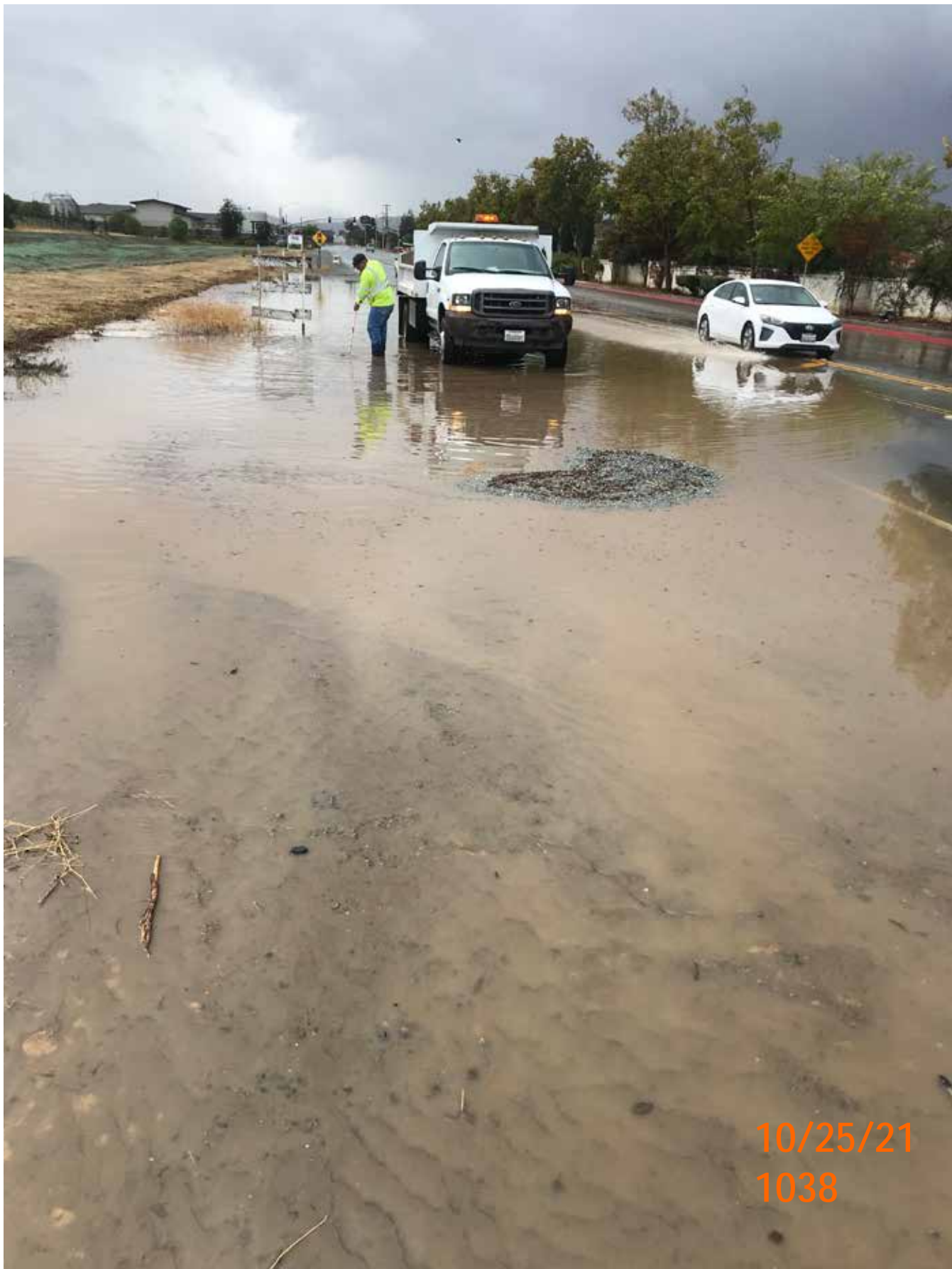
Photo 10. Looking south from edge of pavement on Fairview Rd. Turbid water discharge from Santana Ranch construction site. Sediment in lower half of photo is soil surface east of edge of pavement. City attempting to find and clear storm drain feature.
