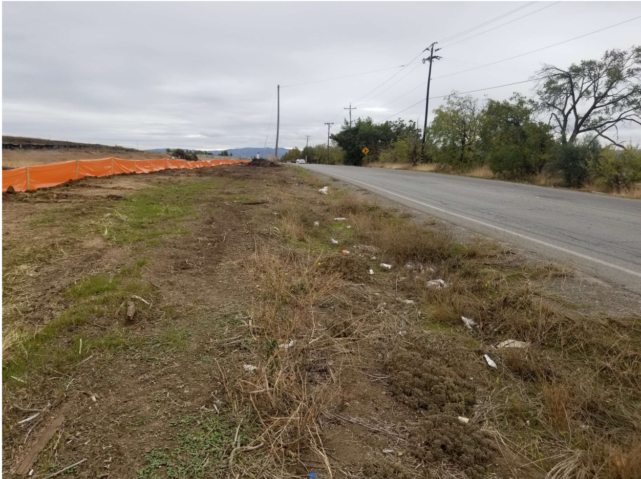
Figure 16. Ditch-52.jpg - Fairview Road east side ditch
