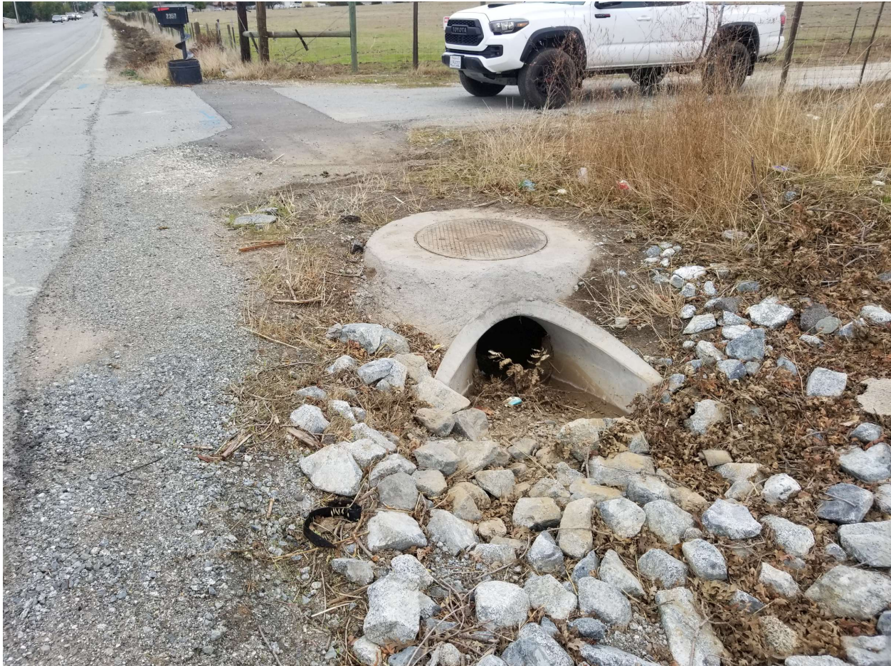
Figure 19. Ditch-56.jpg - Fairview Road east side ditch driveway culvert inlet
