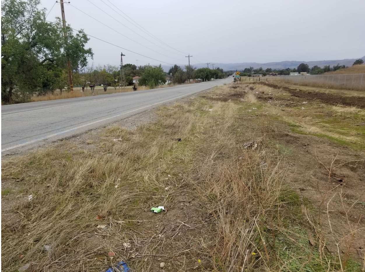
Figure 17. Ditch-53.jpg - Fairview Road east side ditch
