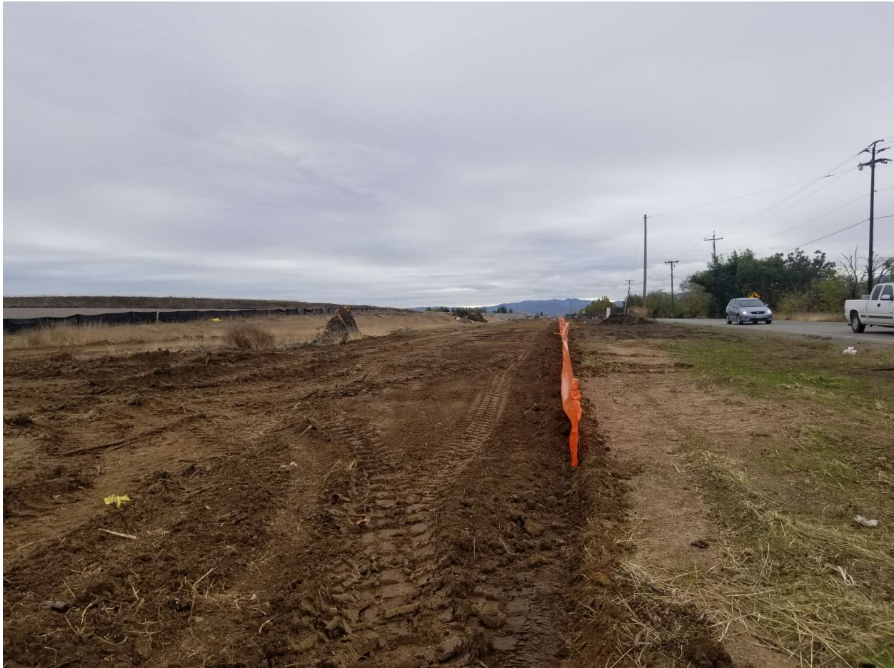
Figure 15. Ditch-49.jpg - Fairview Road east side ditch
