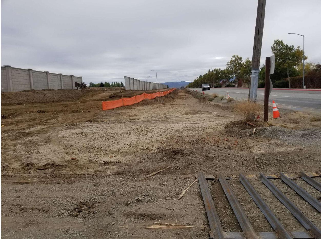
Figure 18. Ditch-54.jpg - Fairview Road east side ditch
