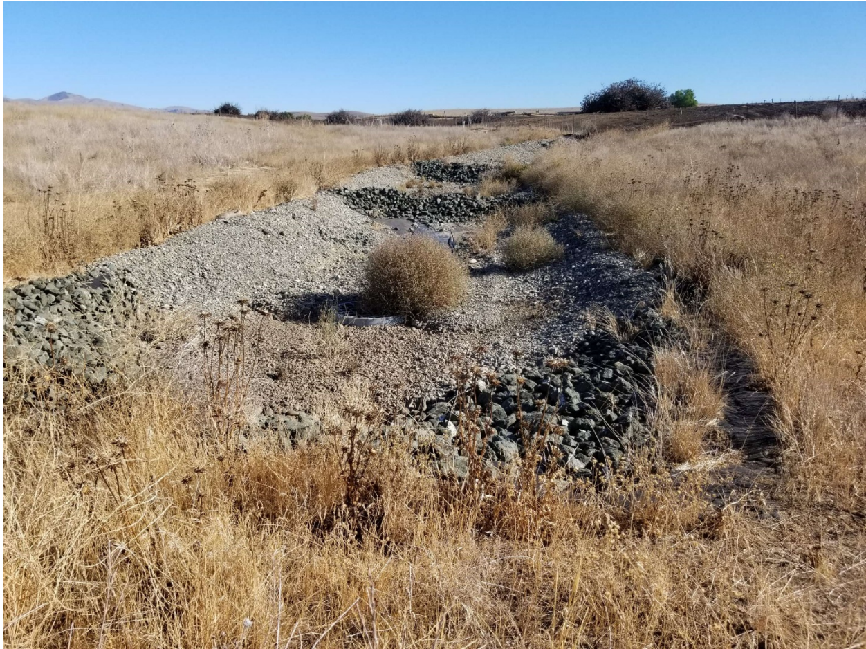
Figure 5. Channel-31.jpg - At inlet to Basin A
