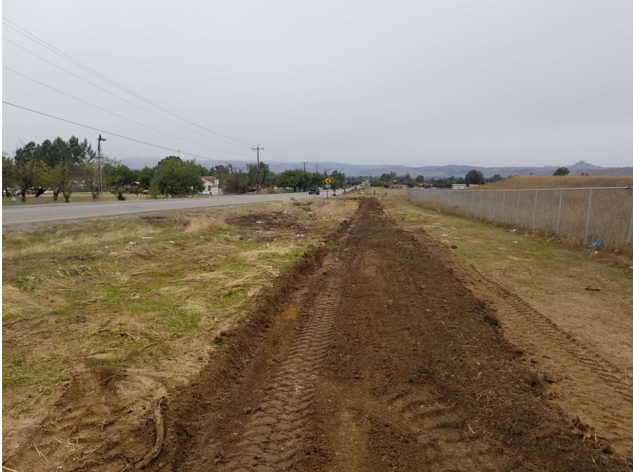
Figure 14. Ditch-48.jpg - Fairview Road east side ditch
