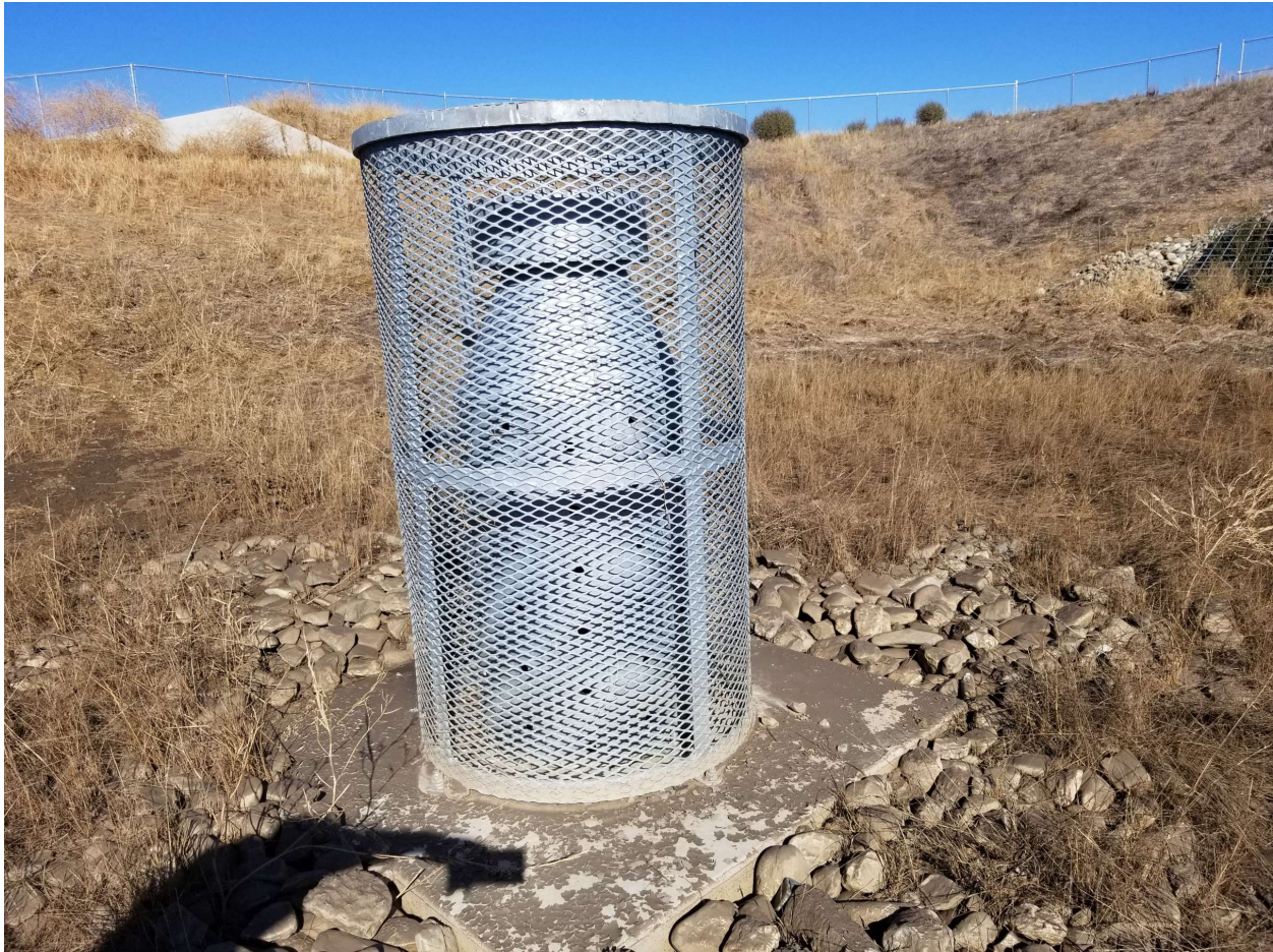
Figure 10. Basin A-23.jpg – Basin A outlet riser
