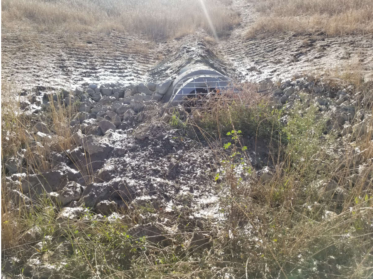
Figure 13. Basin B-41.jpg - Inlet to Basin B partially obstructed
