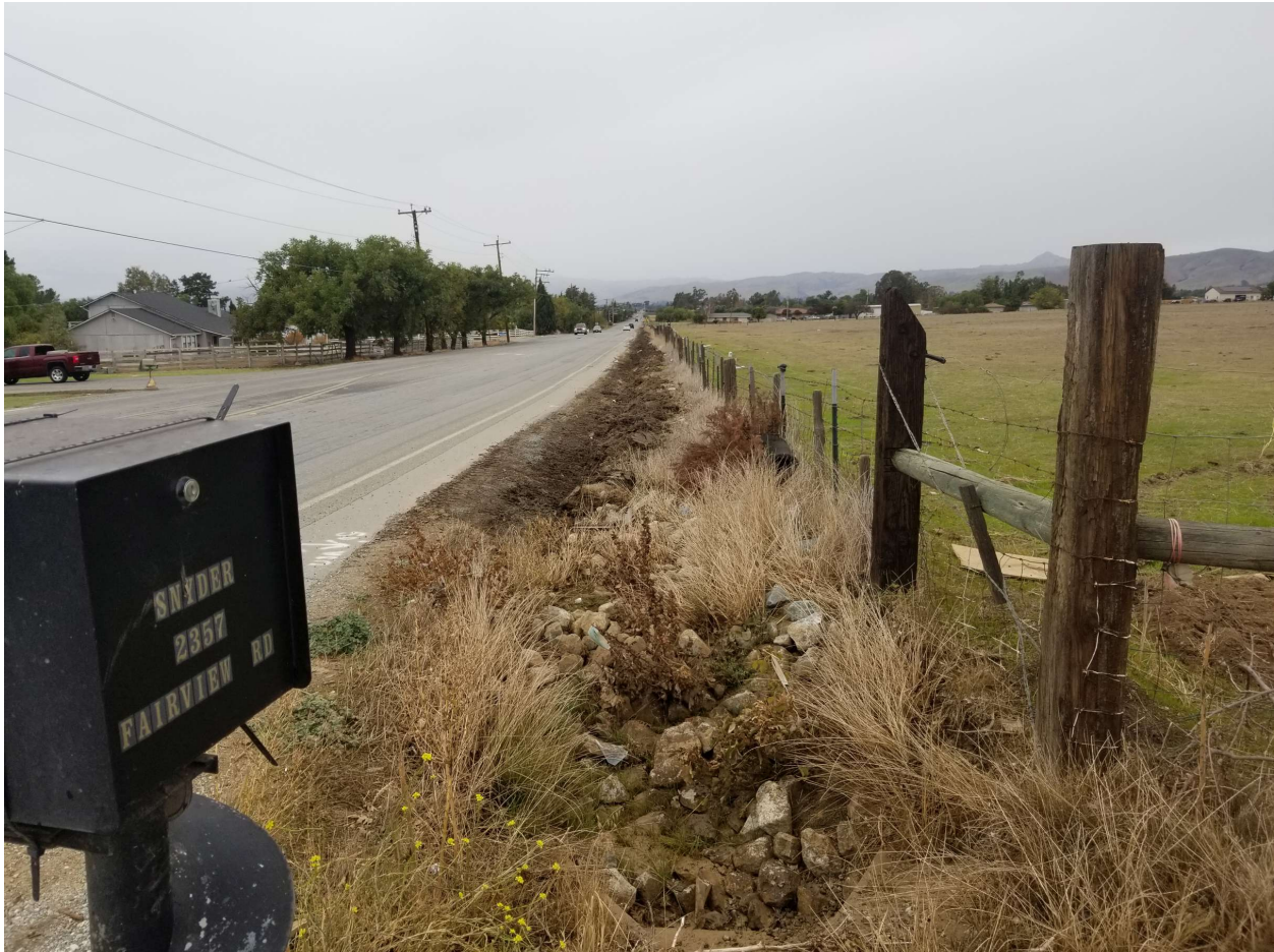
Figure 20. Ditch-58.jpg - Fairview Road east side ditch driveway culvert outlet
