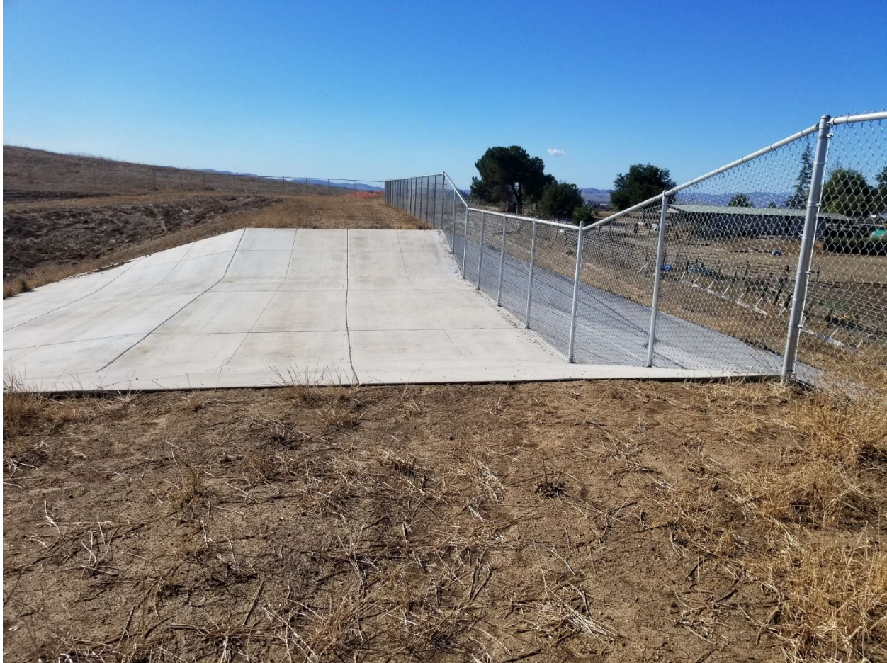
Figure 8. Basin A-17.jpg – Basin A spillway
