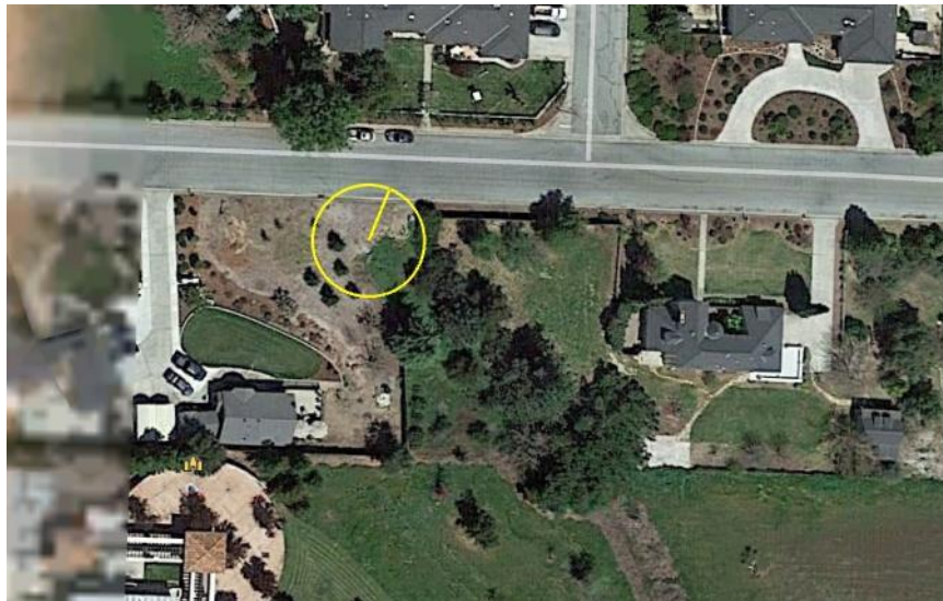
0.05 Acres – Culvert off of Sunset Dr. (Holliday Estates)
